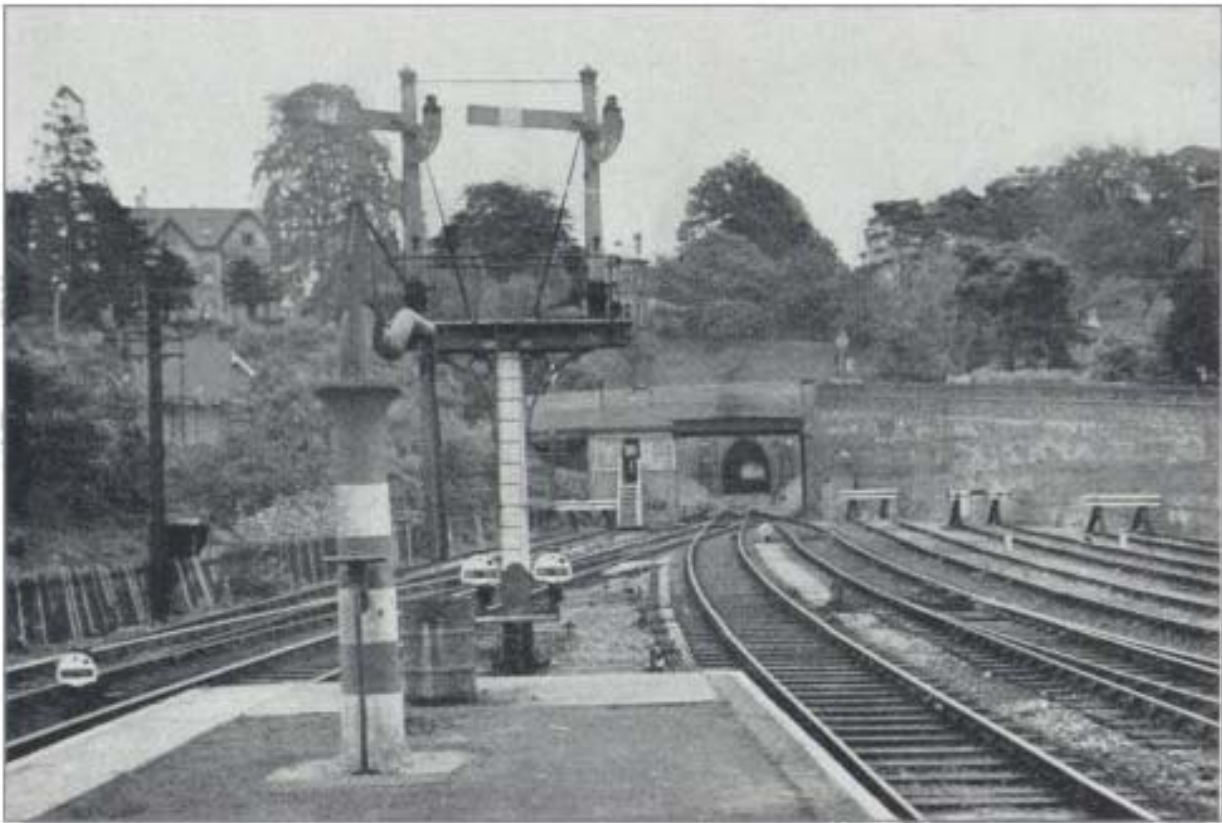
The east end of Tunbridge Wells West Station, looking towards the tunnel
