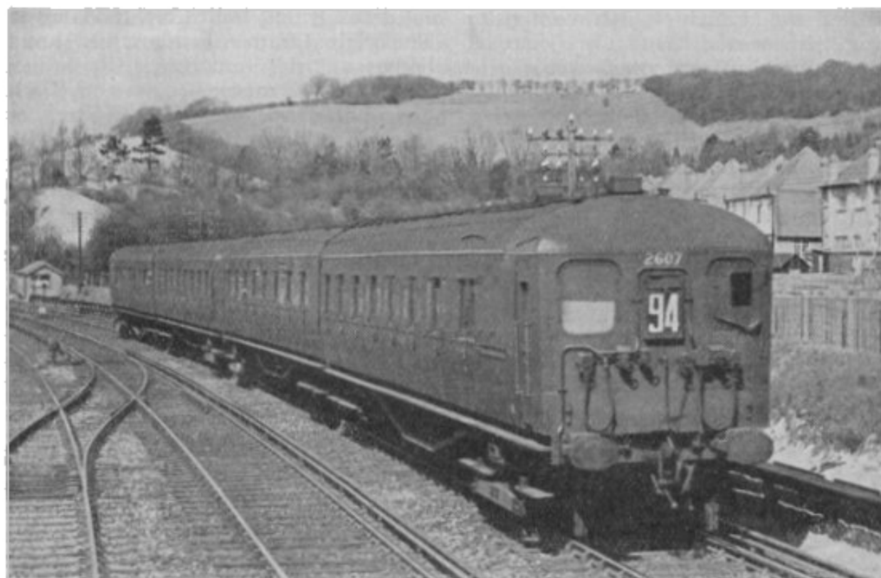
Four-coach stopping main-line train, composed of 2-Hal sets, with wartime modifications
