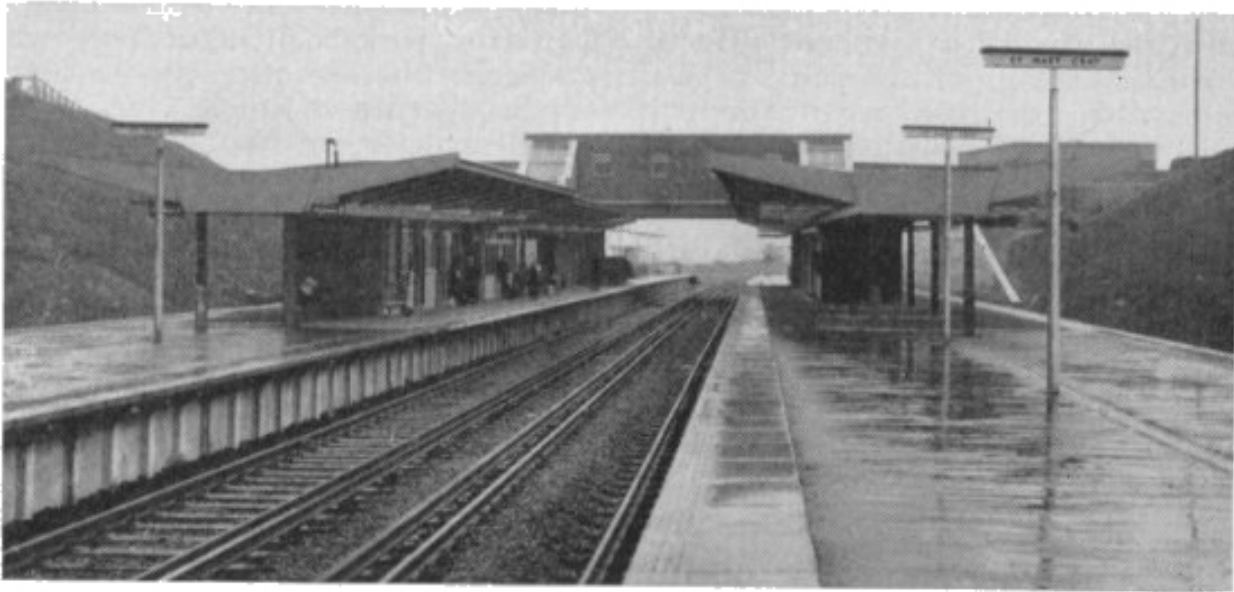
The rebuilt station at St. Mary Cray
