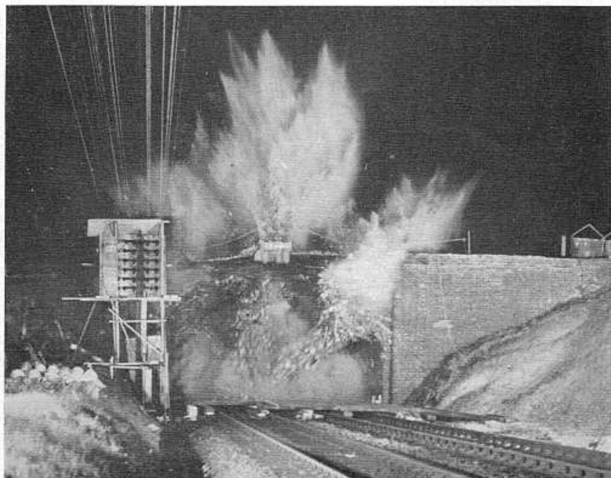
Bridge 179, carrying Quay Lane, being demolished by explosives on November 10. It will be replaced by a new bridge spanning three tracks
