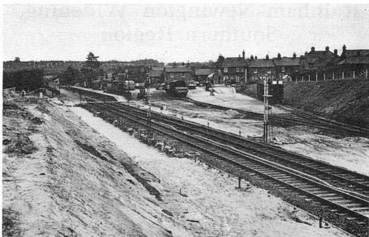
Newington Station from the London end
