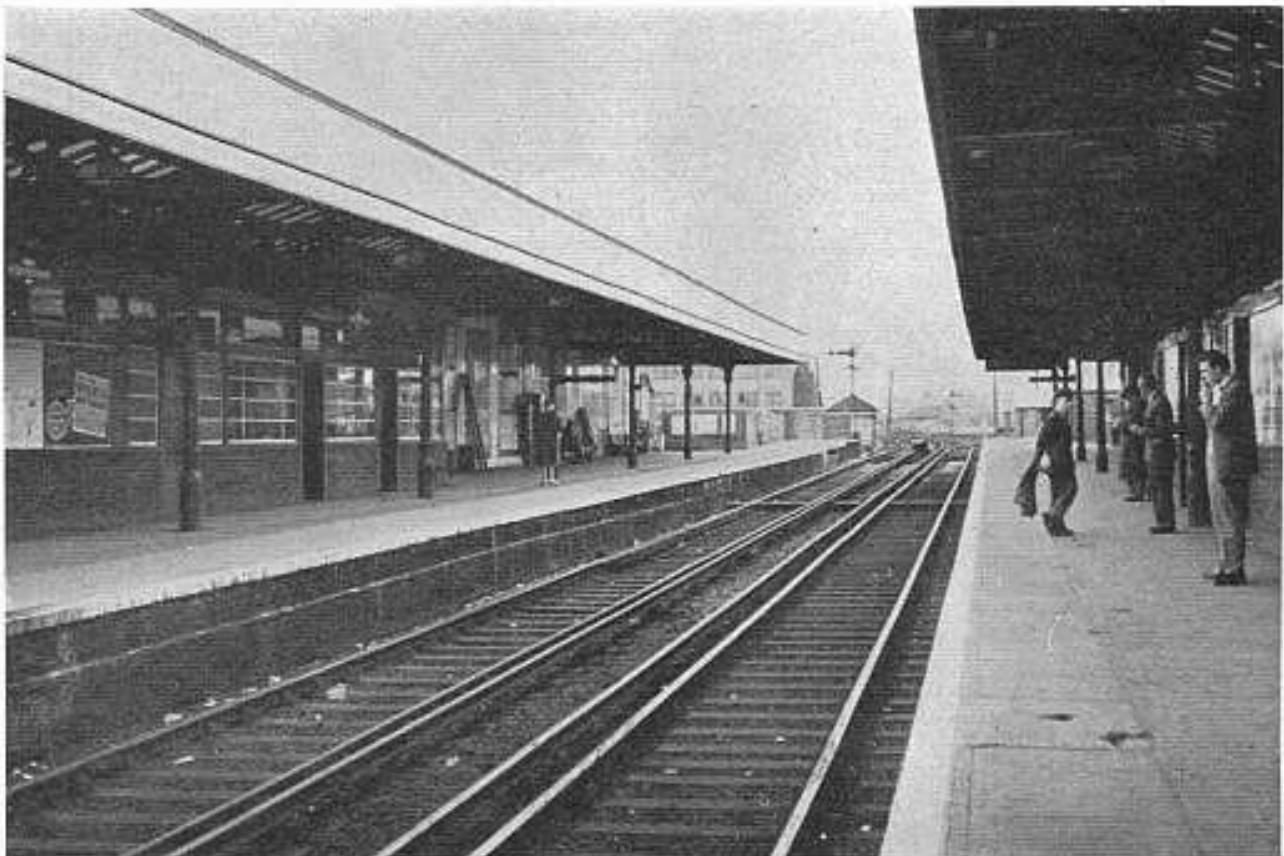
Kingston Station, looking towards New Malden
