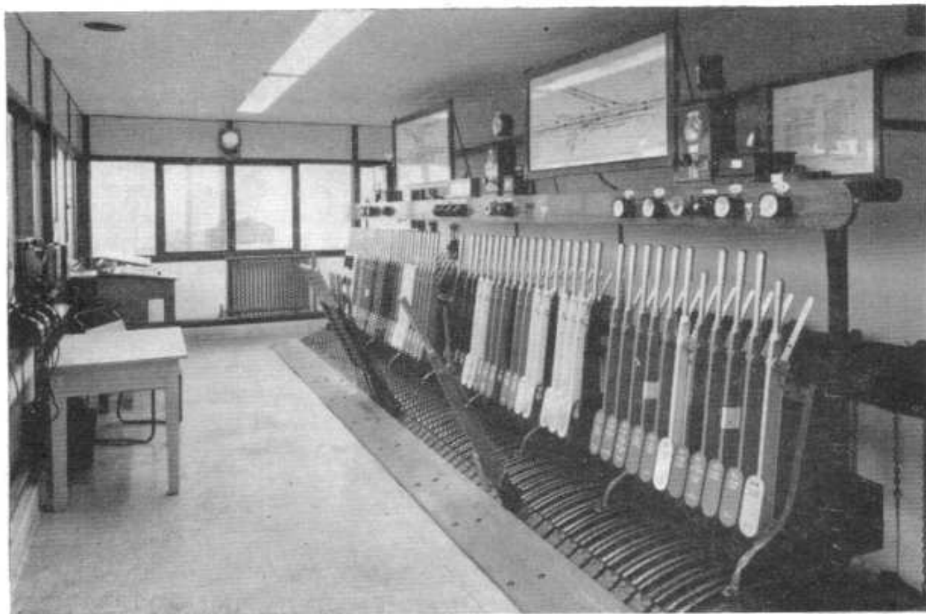
Interior of the new box, showing the lever frame, illuminated diagrams and instruments, with advance indicators set to face the train-booking desk
