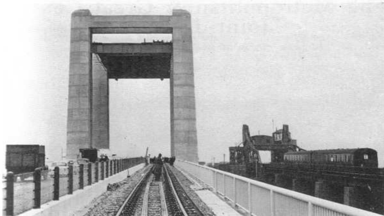
Lifting span of the new bridge in the raised position, showing the rail approach and a train crossing the old bridge
