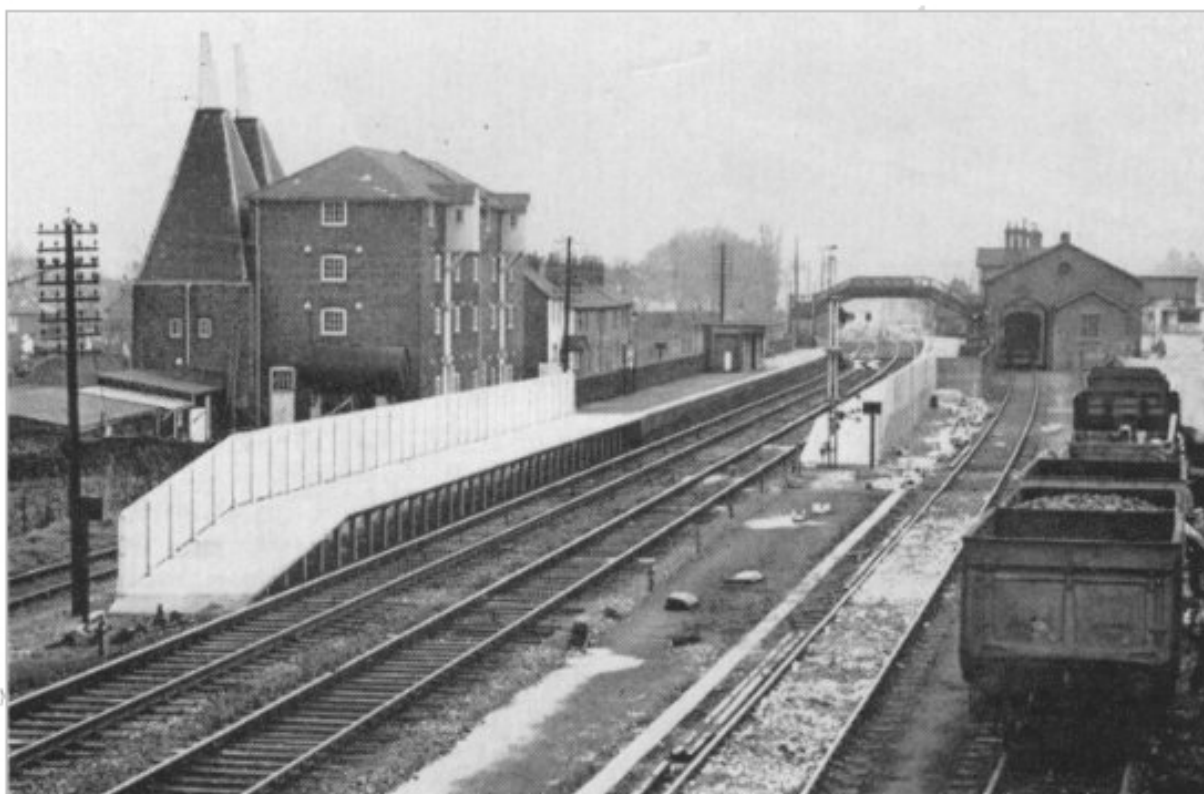
Platform extensions at Rainham to accommodate eight-car trains
