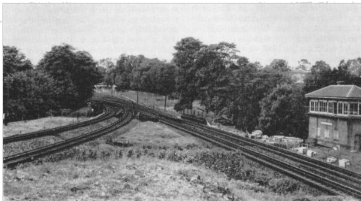
View of Bickley Junction, looking towards London, showing the sharply-curved loops which are to be replaced by improved lines
