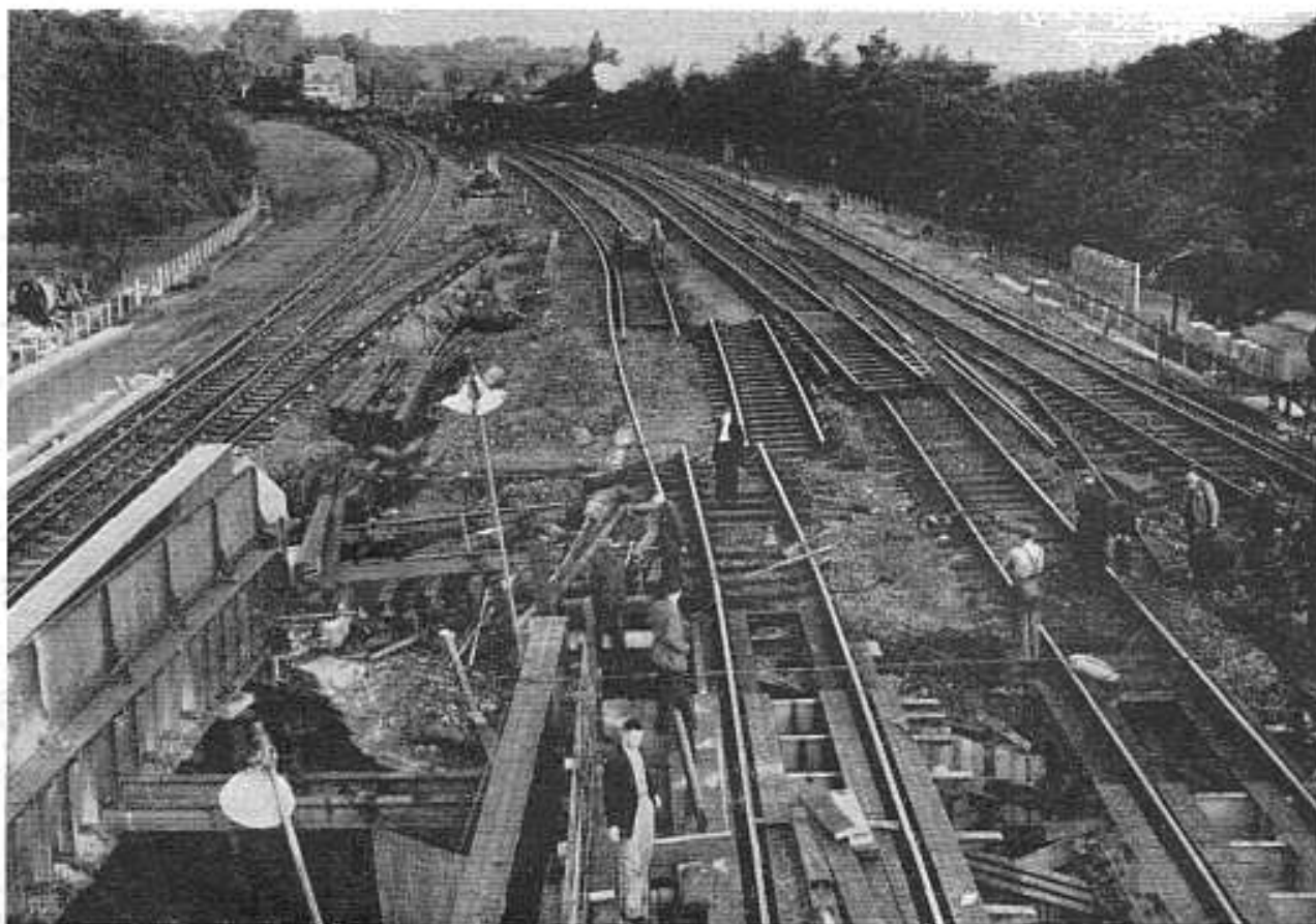
Scene at Shortlands on September 7, 1958, with the up and down fast lines broken for slewing. Switch and crossing work is proceeding in the distance
