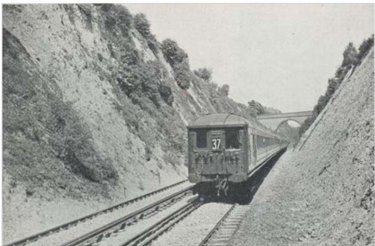
London Bridge-Brighton electric train in the cutting between Star bridge and Merstham tunnel. This section of line was originally part of the Croydon, Merstham & Godstone Iron Railway opened in 1805
