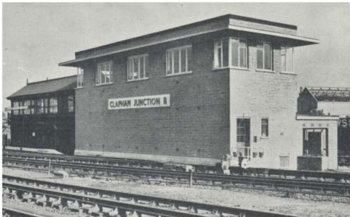
The new Clapham Junction " B " box, which replaces the mechanical box on the left. The old box has now been demolished
